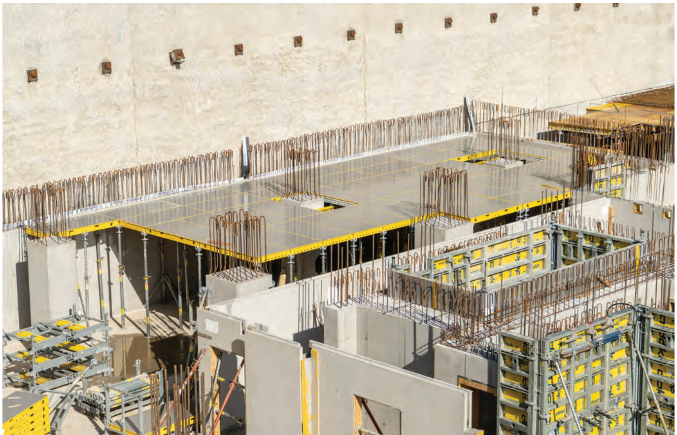
The DokaXdek system in use.
