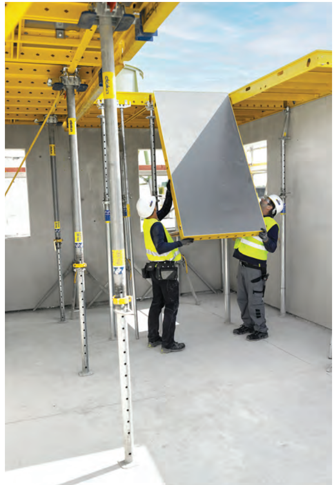
The DokaXdek panel can be assembled and disassembled from the ground, requiring only two people.
