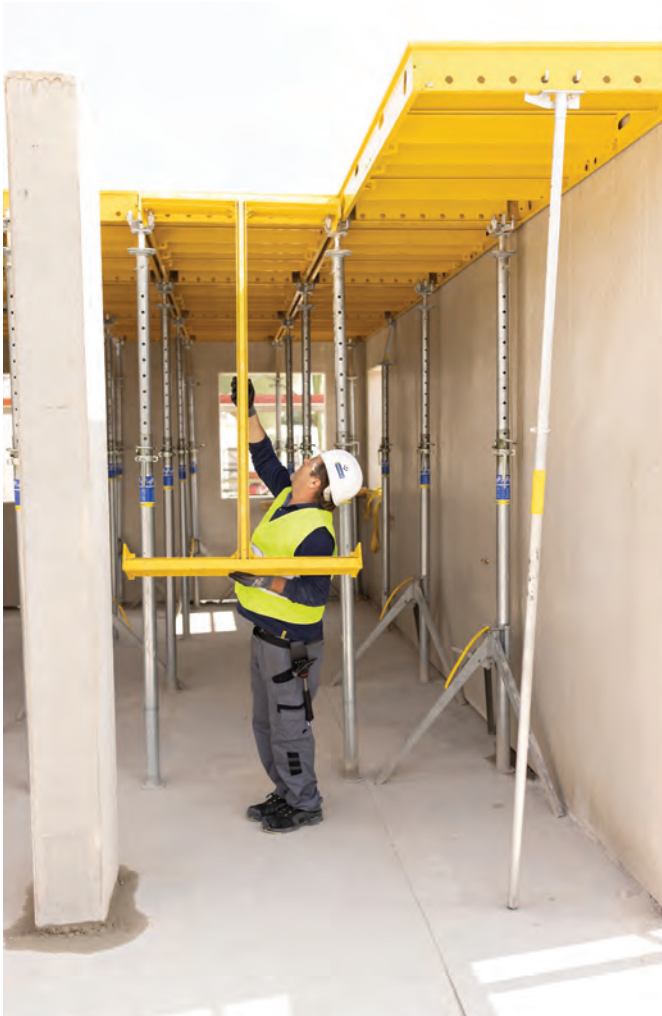
The DokaXdek I-frame can form slabs in a one-person setup.
