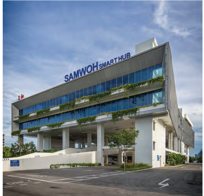
Located in the Sungei Kadut Eco-District, the new Samwoh Smart Hub is the first positive energy industrial building in Singapore. It was built using various types of recycled construction materials.
