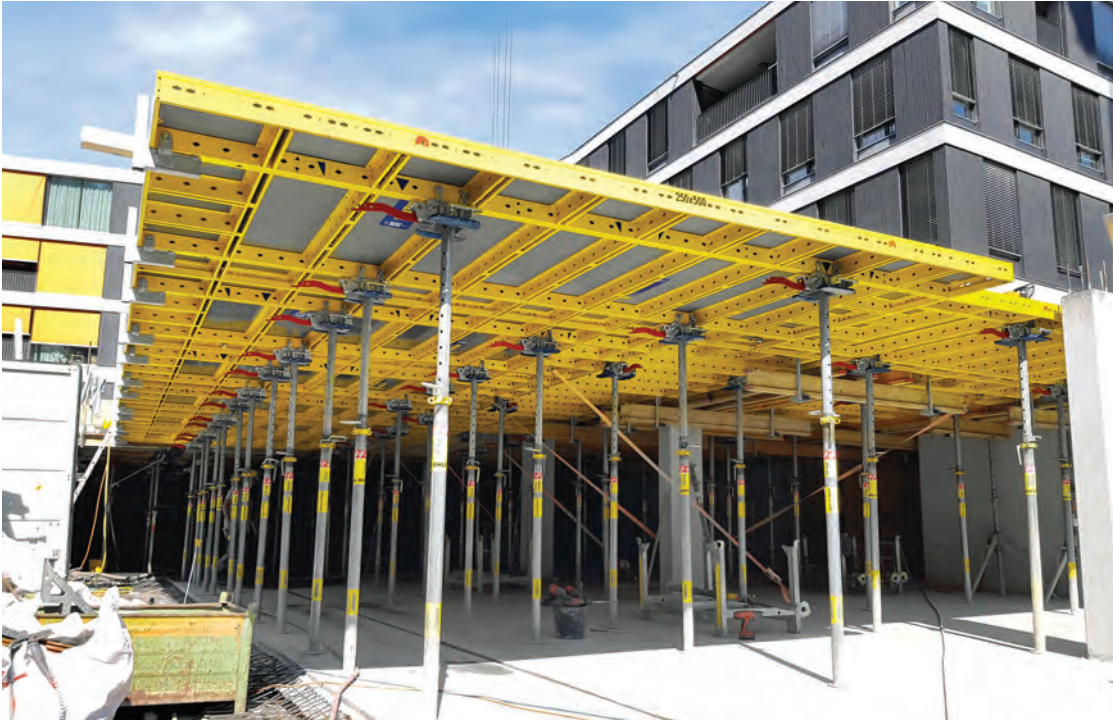
LEFT: The DokaXdek table offers all the usual advantages of a slab table, such as speed, safety and economy – especially on medium to large construction sites.
